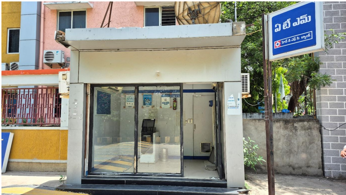
ATM facility at IARE
