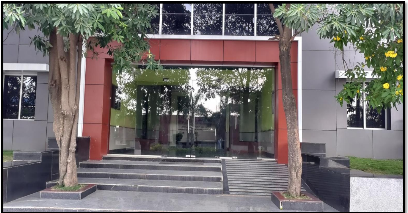
Barrier Free Ramps
