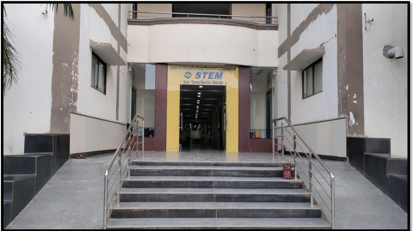
Barrier Free Ramps
